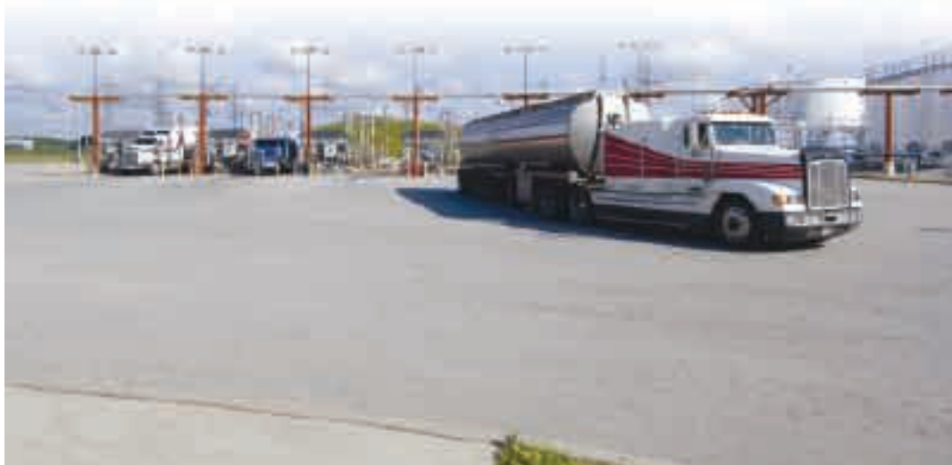
Tank truck load rack facility at Suncor in Canada
