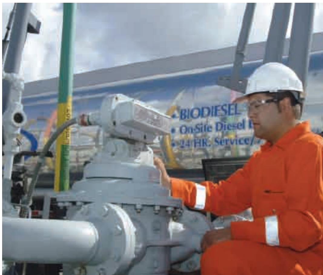
Positive displacement measurement system for biodiesel blending
